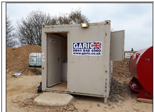
Site cabin, in the south of the site.
